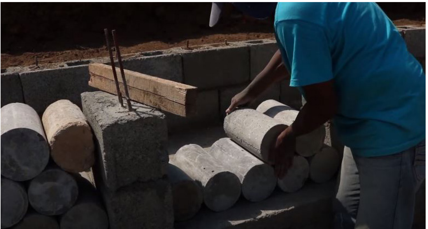
Fig. 8. Assembly process for the modules' perforated covers. Photo: Laura Avila (2019).
