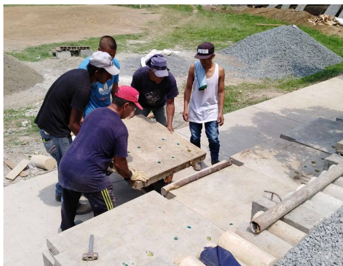
Fig. 6. Assembly process for the modules' perforated covers. Photo: Laura Avila (2019).
